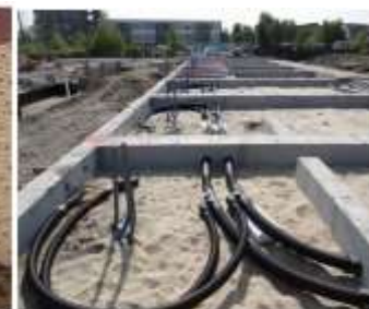
Figure 3: Alkmaar, NL: 8 houses connected to District Heating in 1,5 hrs
