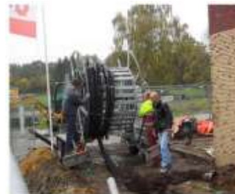
Figure 2: Hengelo, NL: 10 houses connected to the heating grid (2 lines) in 1,5 hrs
